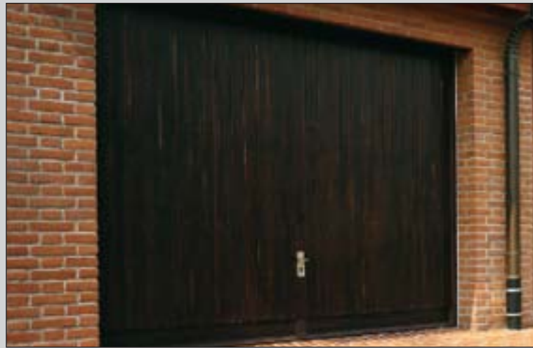
Prior to renovation
