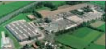
Head Office Verl-Sürenheide Works
